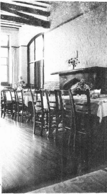
Dining room, Diocesan Training College, Ditchling Road
